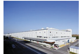
The waterborne paint Plant
