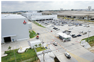
Mitsubishi Motors (Thailand) Co., Ltd. (MMTh)
